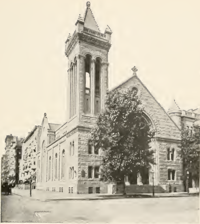
SCOTCH PRESBYTERIAN CHURCH, CORNER NINETY-SIXTH STREET AND CENTRAL PARK WEST, NEW YORK. (1756-1906.)
