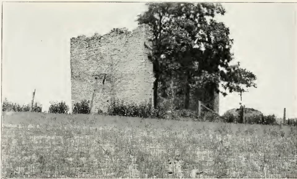
Ruins of Liberty Hall Academy—Exterior View
