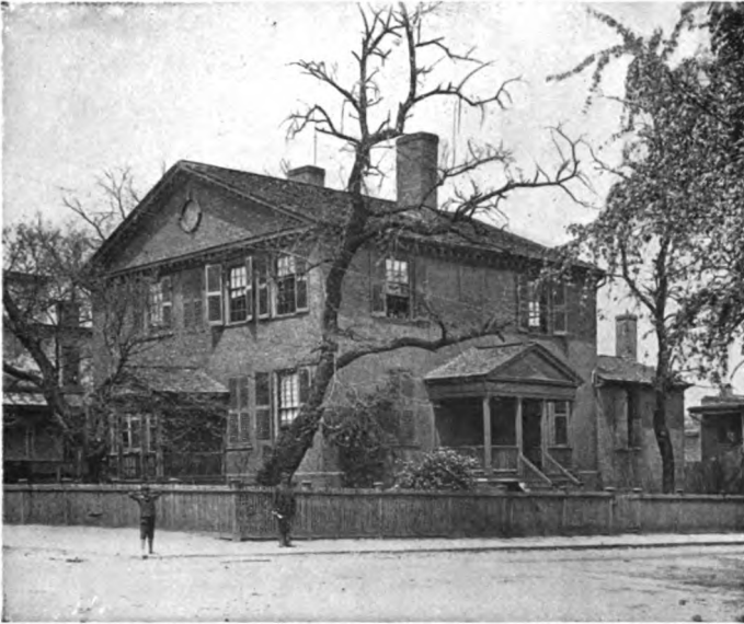
MARSHALL HOUSE, RICHMOND, VA.
