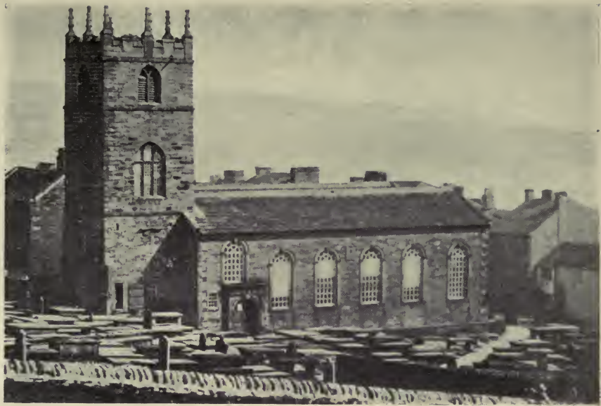
HAWORTH CHURCH BEFORE RESTORATION
