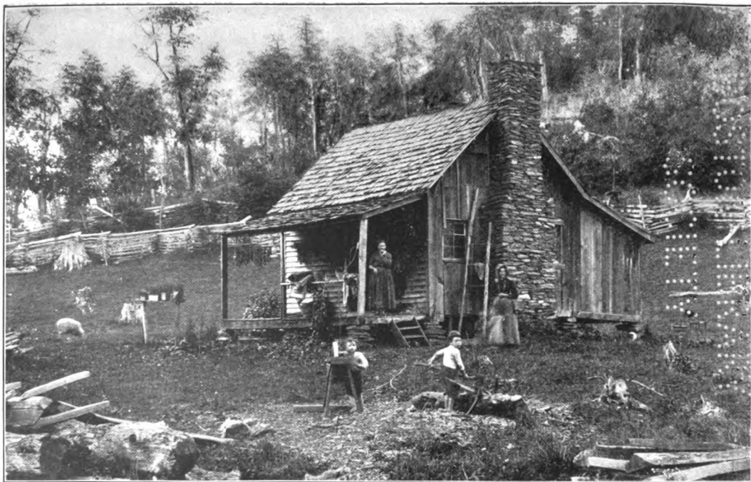
THE MISTRESS OF THE HOUSE STOOD ON THE PORCH.
