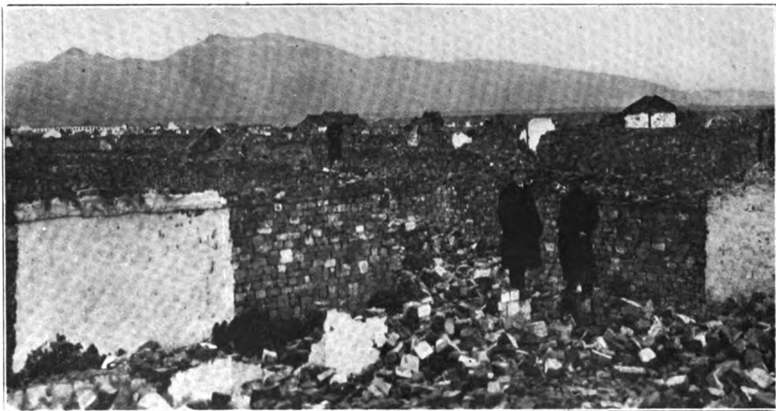
RUINS OF THE MANCHU QUARTERS, NANKING
