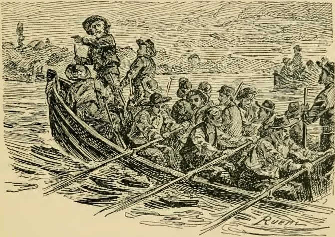
JOHN BROWN CROSSING THE RIVER INTO VIRGINIA
