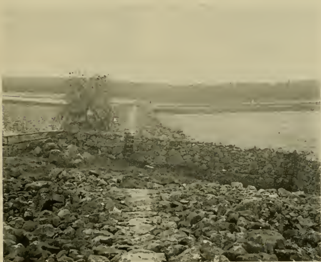
Consumption Dyke at Kingswells
