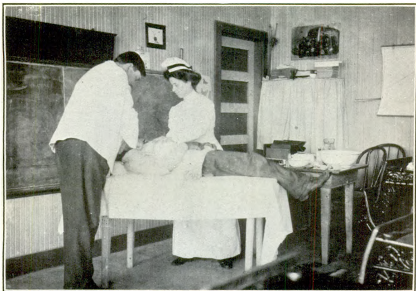
A. CLINIC IN SCHOOL ROOM.
