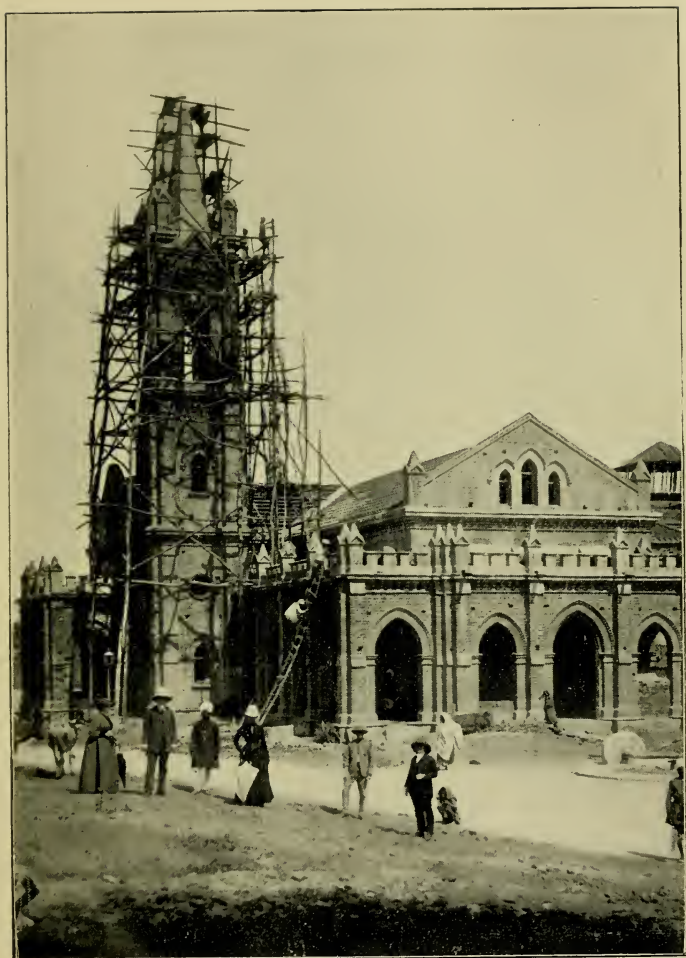
CHURCH IN COURSE OF ERECTION.
