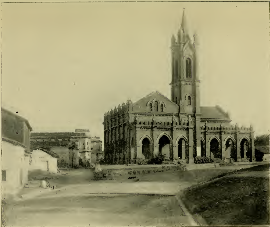
CHURCH AND READING-ROOM COMPLETED.
