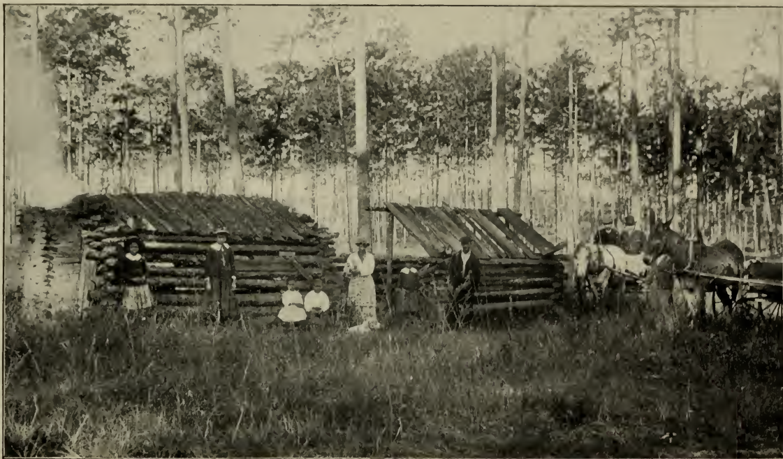
NEGRO CABINS IN THE PINE WOODS OF FLORIDA.
