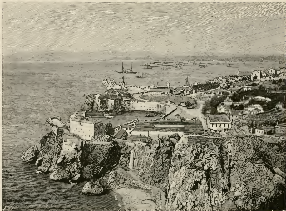
THE NEW MOLE AND ROSIA BAY,
