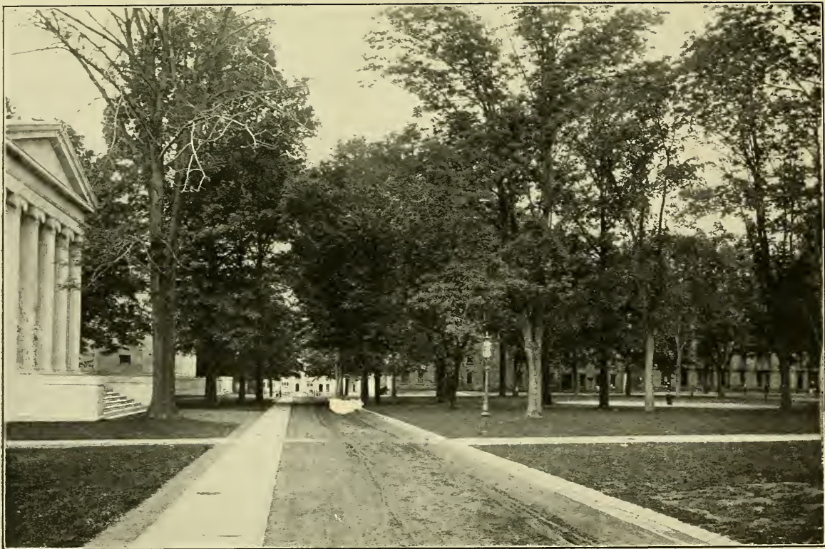
View towards the West.
