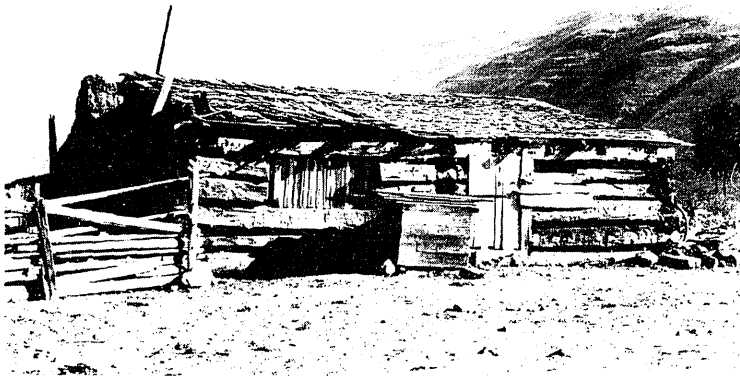
The Spalding mission house, erected in 1838, as it appeared about 1890. The upper part has been removed. The notches in the top log where the cross beams were laid can be seen. The view is toward the southeast. Today the North and South Highway runs just east of this location.
