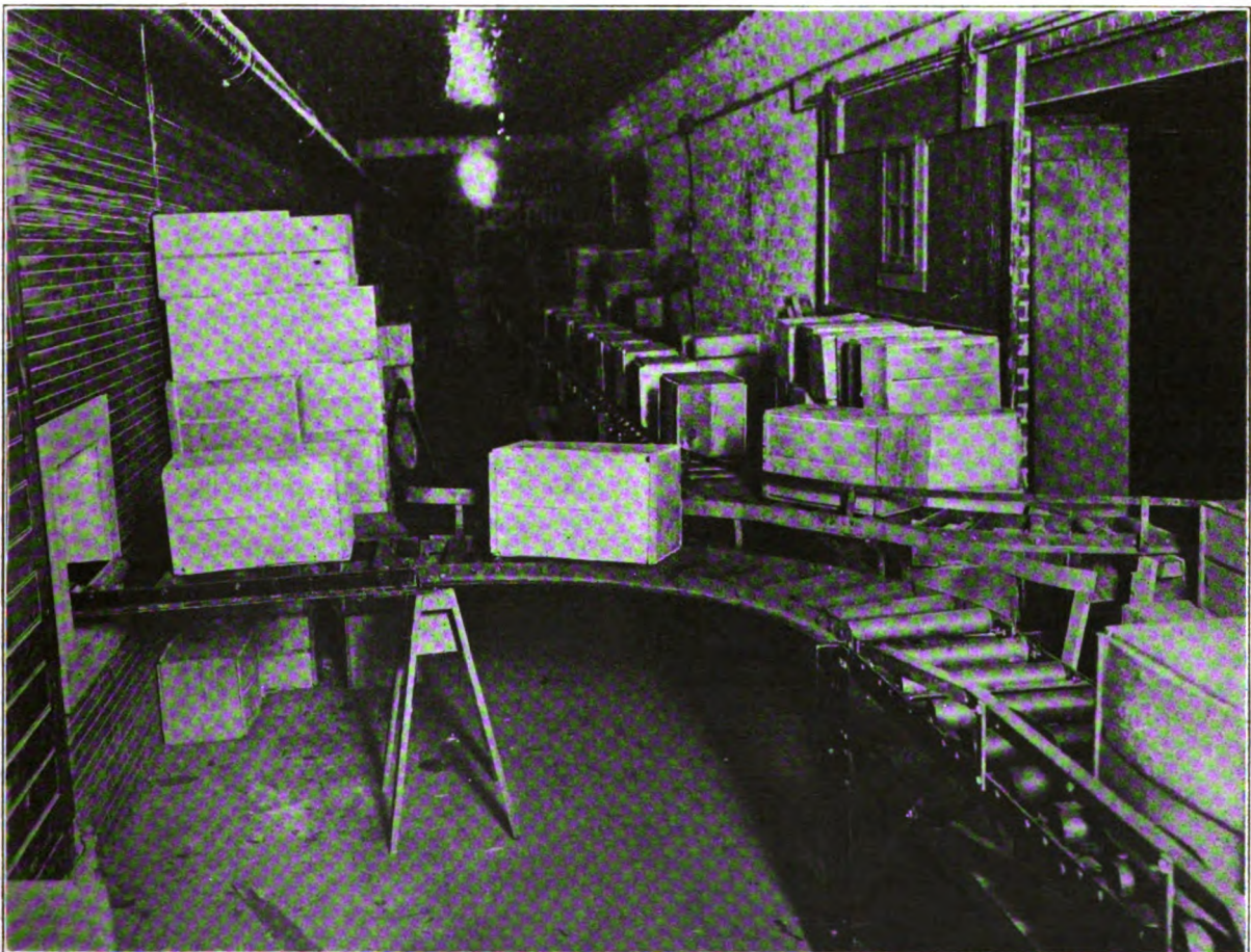
Conveyor System on First Floor of Warehouse
