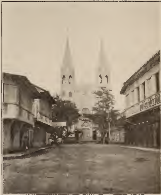
SAN SEBASTIAN R. C. CHURCH, MANILA Made in France and shipped in sections to Manila
