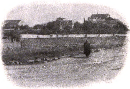
MISSION BUILDINGS, LATAKIA, SYRIA From left to right—Boys' School, Hospital, Girls' School
